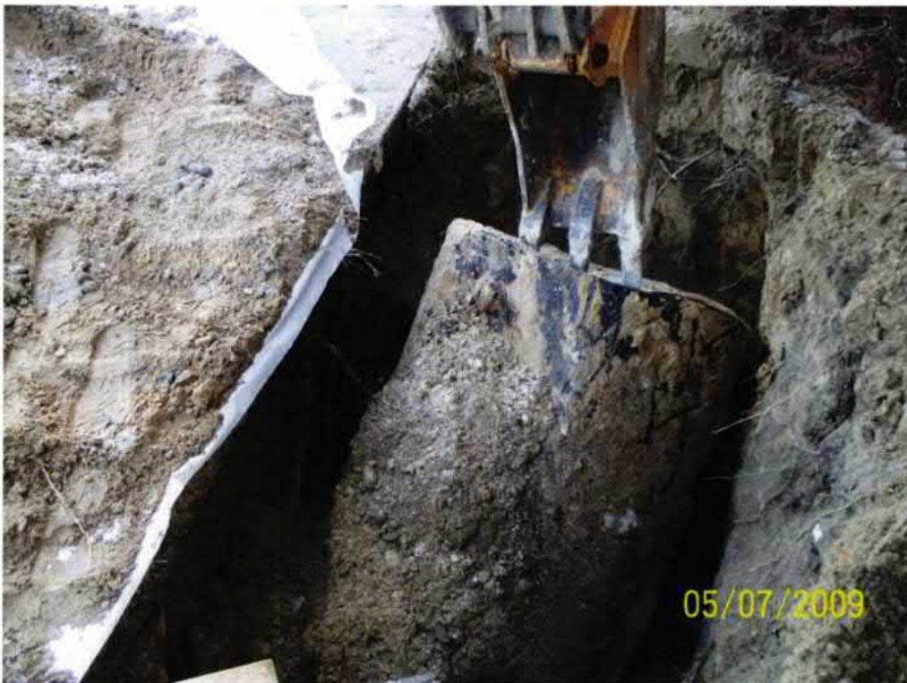
Picture 2: UST 1000Bobwhite Drive being removed from the excavation.
